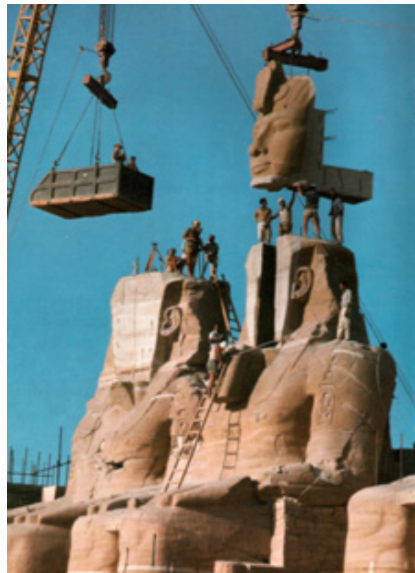
Moving of the Abu Simbel temple, threatened by the construction of the Aswan Dam (Egypt, 1967)
